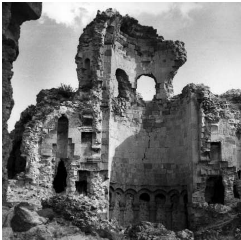
27. Cathedral of Bana. Interior looking east, as in 1970s
