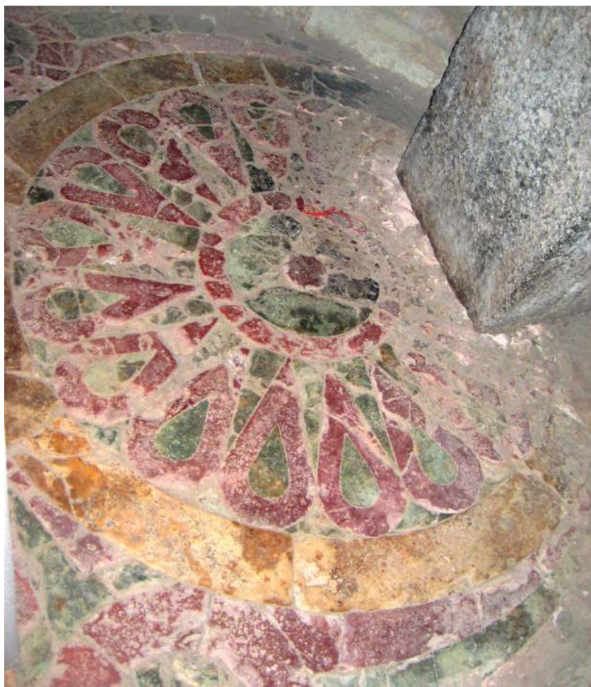
63. Cathedral of Ruisi, northern chapel. Floor
