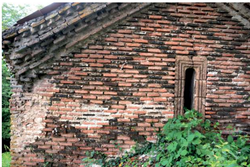
79. Sanagire Church. Western façade, detail of brickwork
