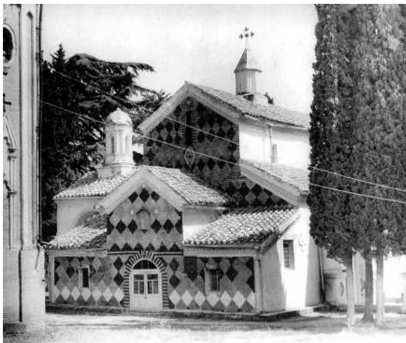
80. Church of St George in Bodbe Monastery. Western façade, as in 1970
