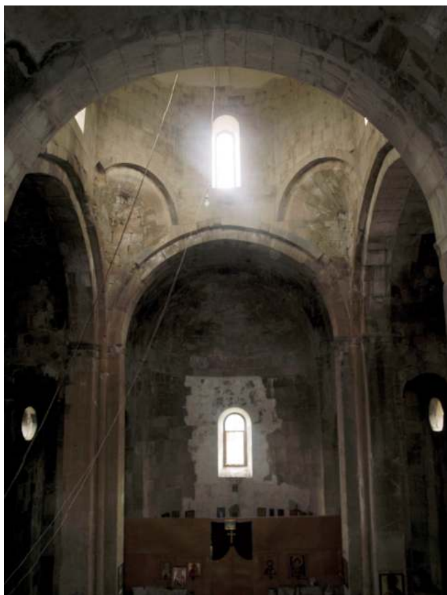
24. Tsromi Church. Interior looking east
